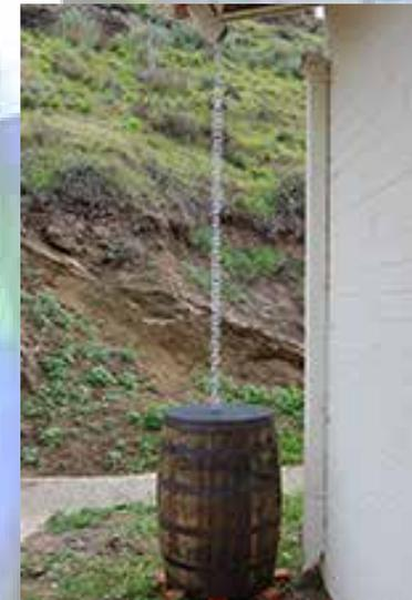
Rain Barrel using a Chain
